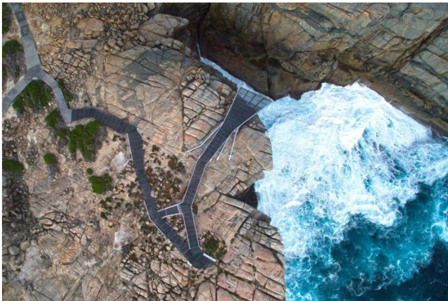
Photo 2: Aerial view of the walkway and platform at The Gap 7
